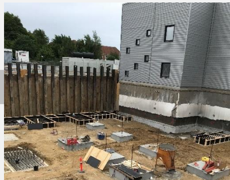
Construction of fill/finish plant
