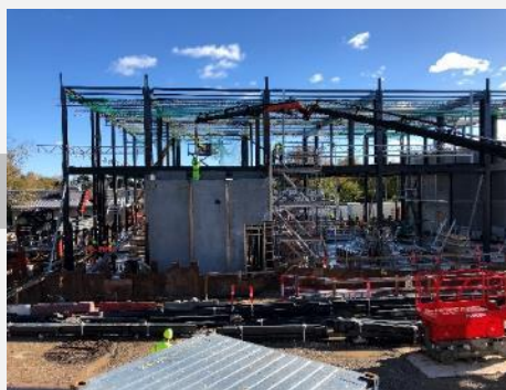
Construction of fill/finish plant
