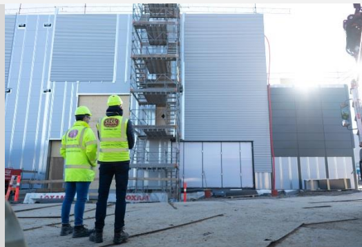
Construction of fill/finish plant
